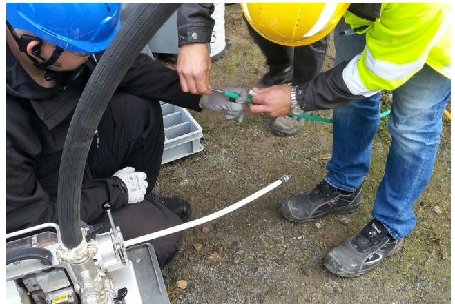
Inserting a sonde into a micro duct before connecting duct to a jetting machine.
