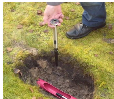
Exact location of the sonde and duct saves unnecessary digging.
